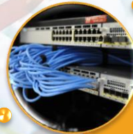
STORAGE MANAGEMENT SYSTEM
