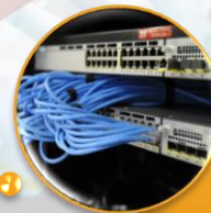
STORAGE MANAGEMENT SYSTEM
